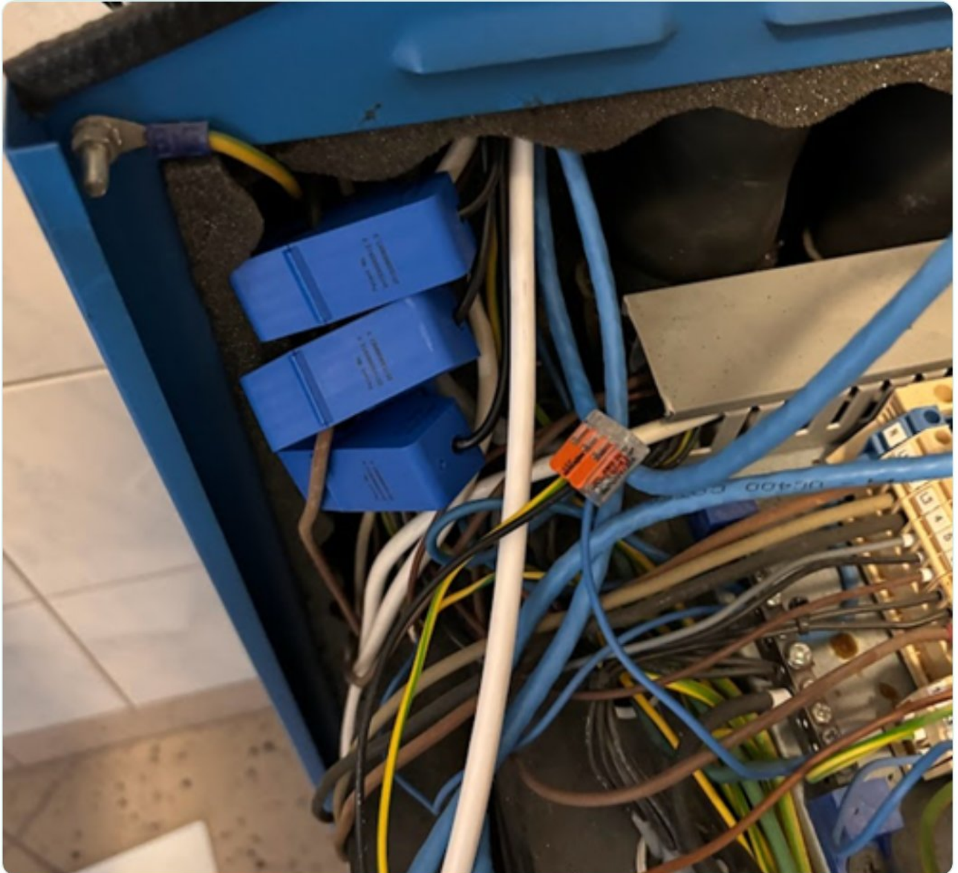
Current sensors on the phases L1, L2 and L3
