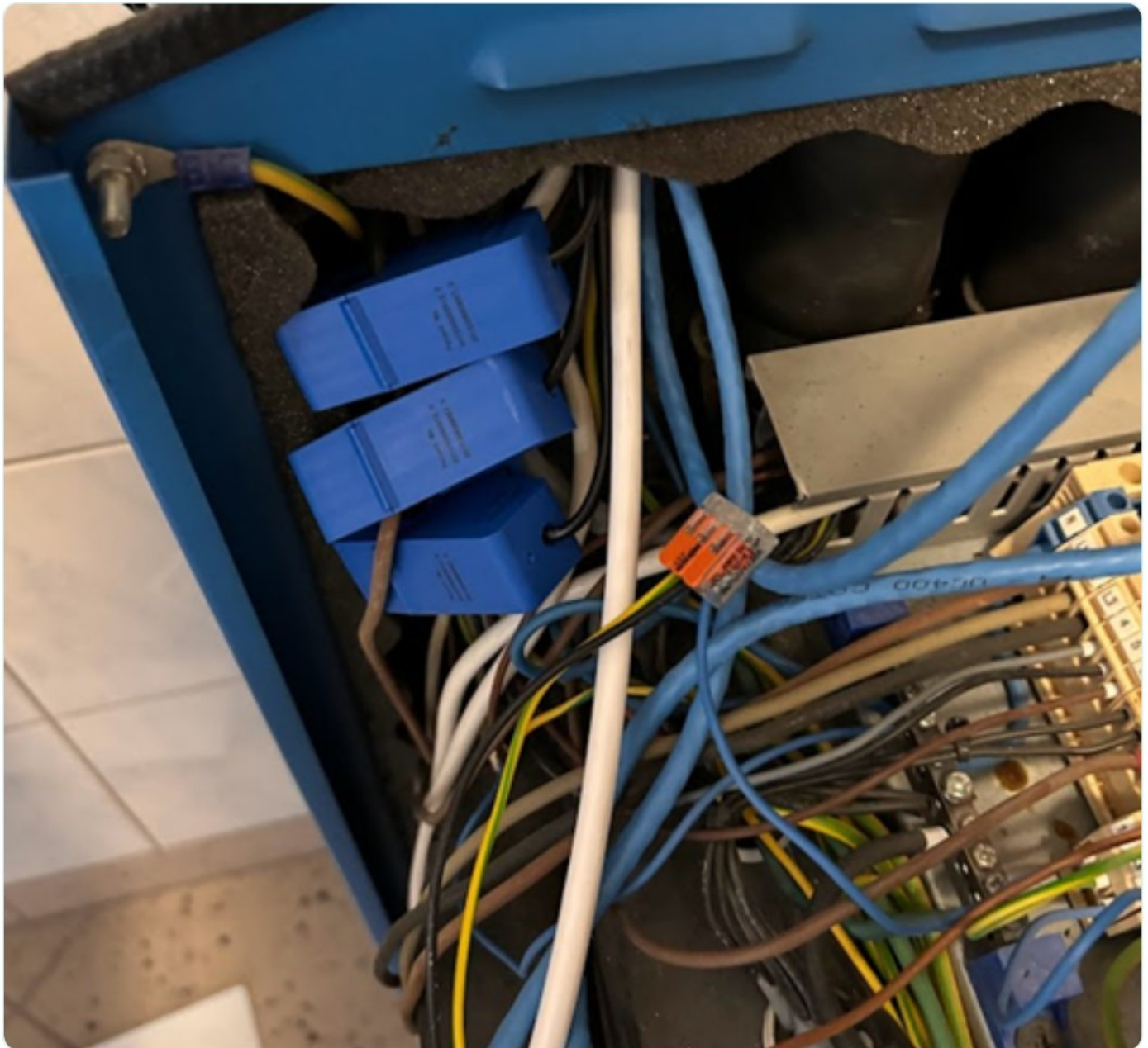
Current sensors on phases L1, L2 and L3
